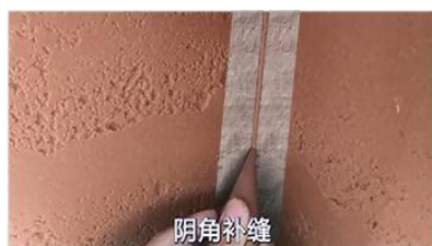
7、Fill the internal corners with caulk
