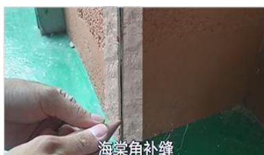
8、Fill the external corners with caulk
