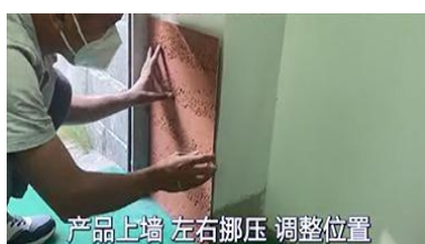
2、Glue the back of the product onto the wall
