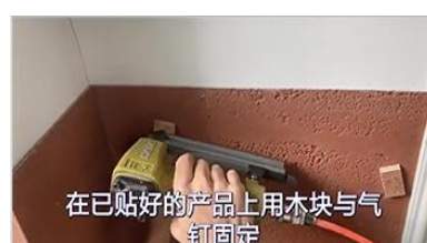
3、Fit it with air nails
