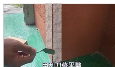
9、Use a scraper to smooth the caulk
