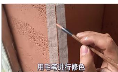
11、Use a color modifier to repair the surface color
