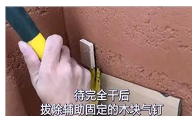
12、After it is completely dry, pull out the air nails
