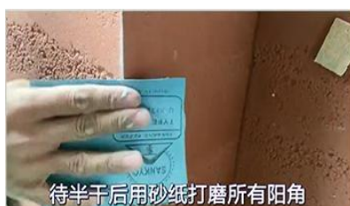
10、Grind the edges and corners
