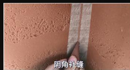
7、Fill the internal corners with caulk
