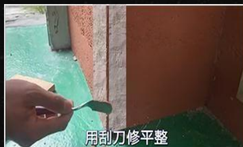
9、Use a scraper to smooth the caulk
