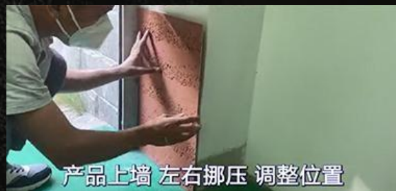
2、Glue the back of the product onto the wall
