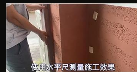
4、Measure the construction size with a ruler
