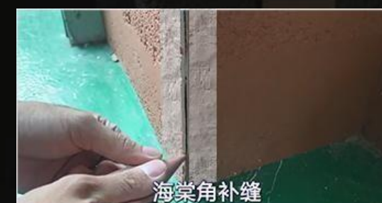
8、Fill the external corners with caulk
