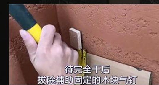
12、After it is completely dry, pull out the air nails
