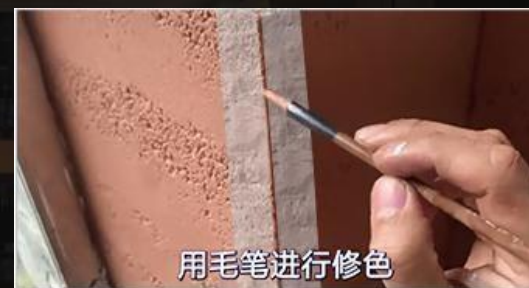
11、Use a color modifier to repair the surface color
