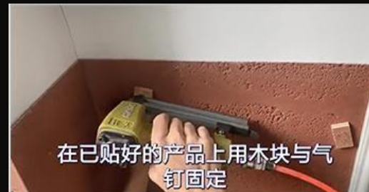
3、Fit it with air nails
