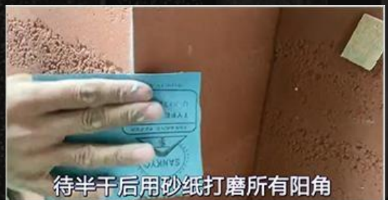
10、Grind the edges and corners
