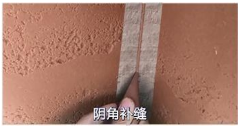
7.阴角填缝 Fill the internal corners with caulk
