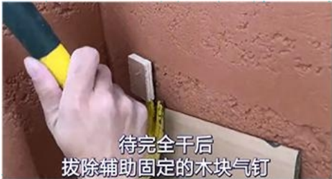
12.待完全干后拔出气钉 After it is completely dry, pull out the air nails
