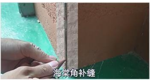
8.阳角填缝 Fill the external corners with caulk
