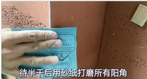
10.打磨 Grind the edges and corners
