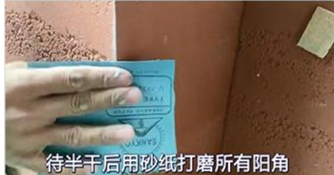
10.打磨 Grind the edges and corners
