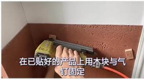
3.用气钉固定 Fit it with air nails
